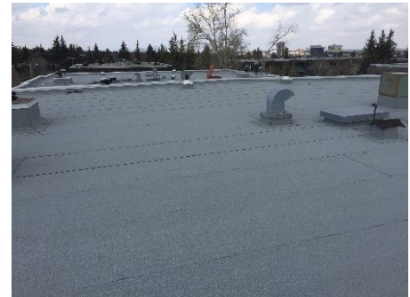
Photograph 18: Typical SBS Roof
