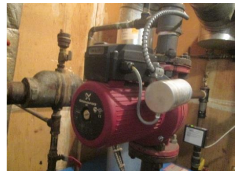
Photograph 23: New Heating Pump
