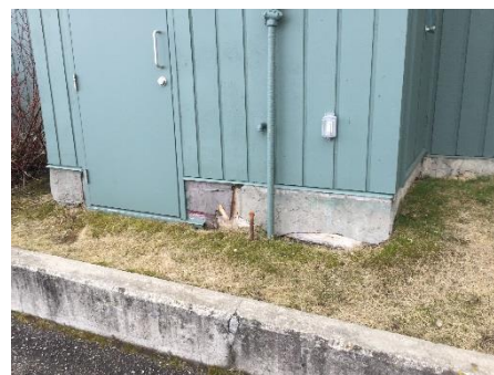
Photograph 11: Delaminated Parging
