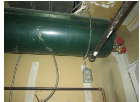
Photograph 25: Expansion Tank
