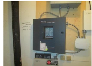
Photograph 32: Typical Fire Alarm Panel
