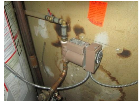
Photograph 29: Domestic Hot Water Recirculation Pump
